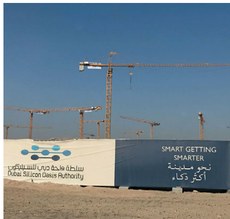
■ With so many cranes being used, the project is making use of Potain's anti-collision technology.
