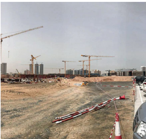
■ Crane supplier, NFT, is said to be the world's largest owner of the French-made Potain cranes.
