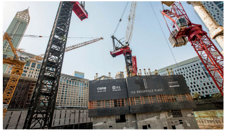
■ Luffing jibs can provide more flexibility on congested sites.
